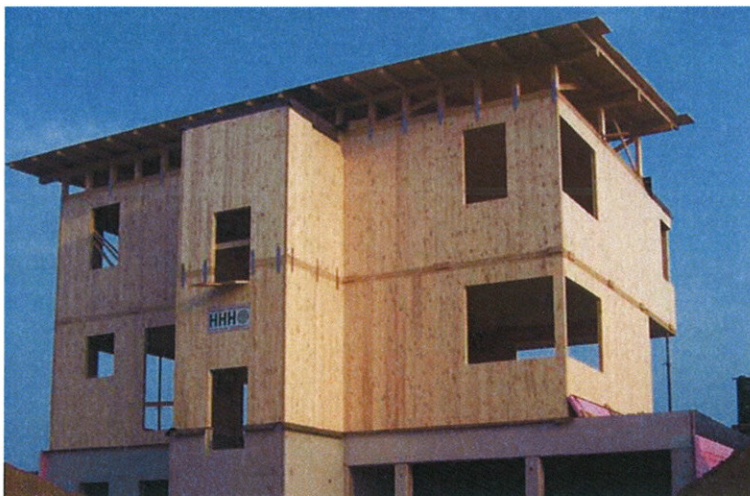
Fig. 1 Example for residential building made of clt-elements as wall and ceilings.
