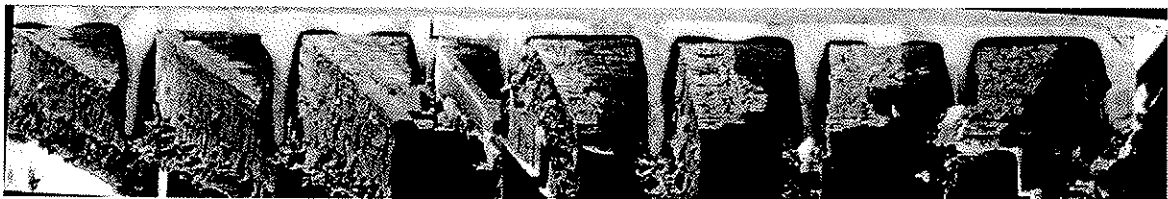
Figure 3 Residual cross-section of a timber slab after 40 minutes ISO-fire exposure; the thin vertical timber members have been exposed to fire on 3 sides, leading to very irregular residual cross-sections
