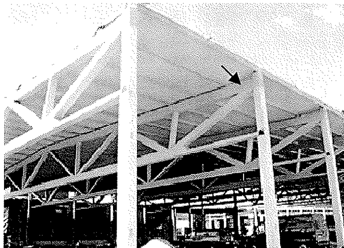
Figure 2. Photograph of the failed roof in Jyväskylä. The arrow shows the joint where dowels were lacking.
