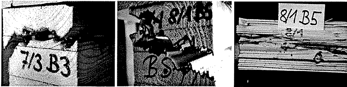
Fig. 10 Failure caused by tension perpendicular to the grain between the upper flange and the web
