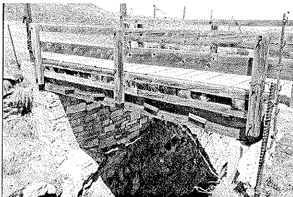
Figure 1: Flitch beam
