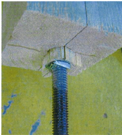
Figure 2: failure mode for axial load
