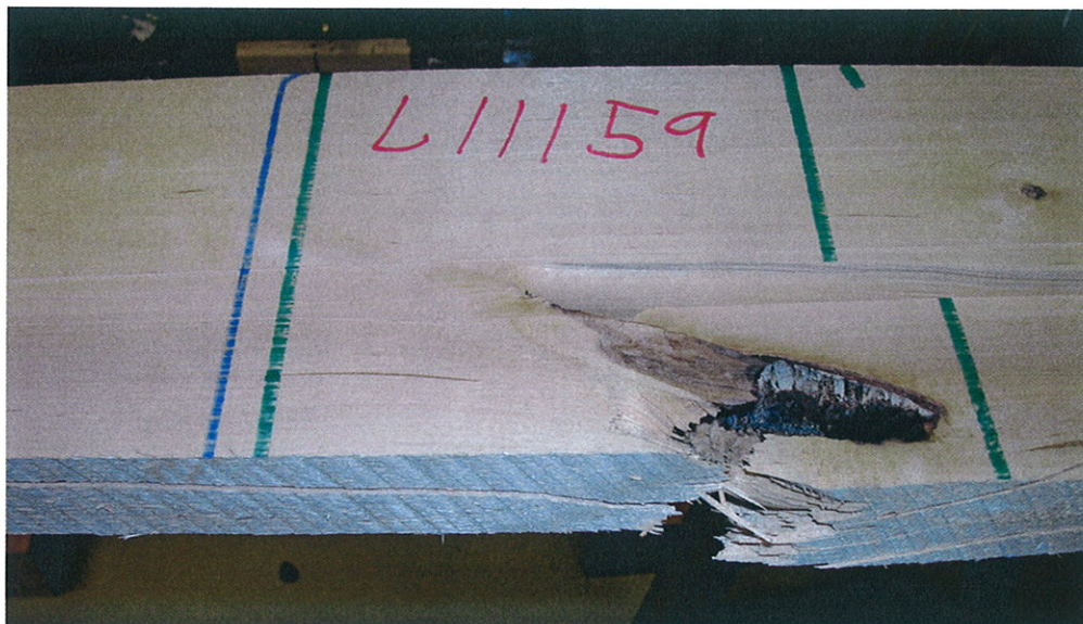
Figure 3. Tension failure at Critical Section in lamination no. L11159 (36 mm x 153 mm) Tension stress at failure: f_{t,0} = 57,2 \text{ N/mm}^2
