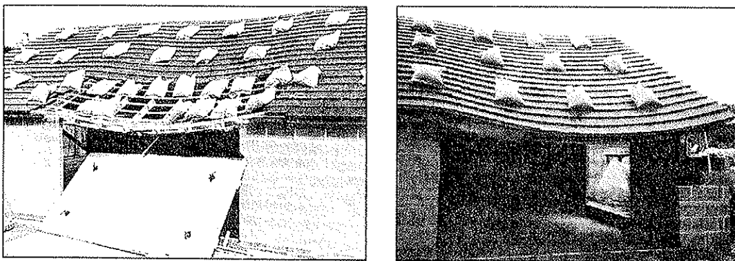
Figure 5 Robustness of Low-Rise Timber Construction [16]
