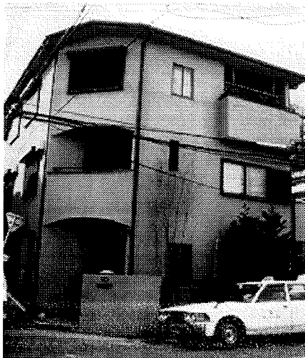
Photo.11- Three story conventional wooden house without damage. Well designed houses had no or few damages.
