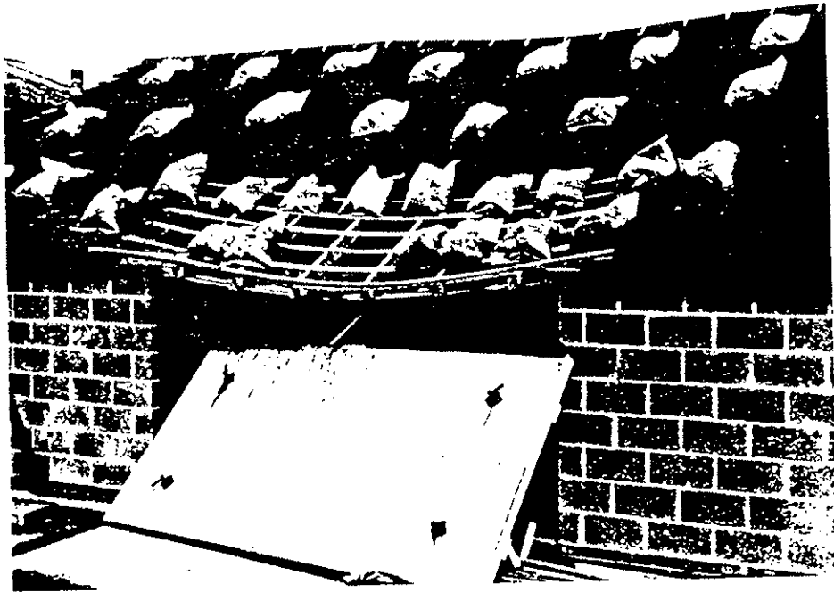
Figure 5 Static position of roof after simulation 4
