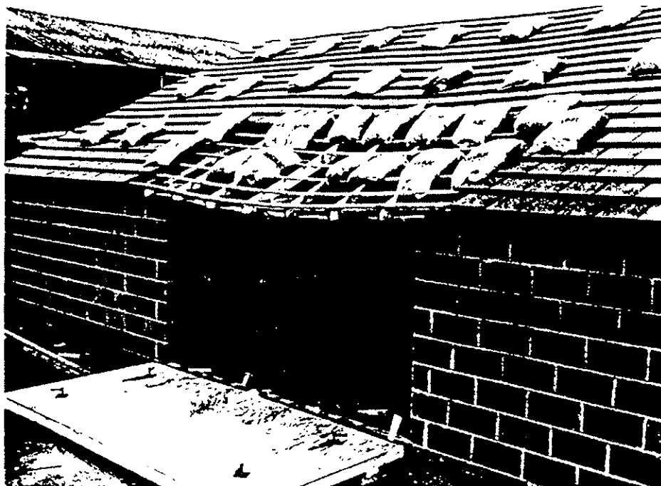
Figure 4 Static position of roof after simulation 2
