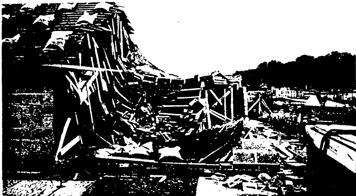
Figure 8 Final collapse of roof, after simulated "accident" to gable end (simulation 6, step 4)
