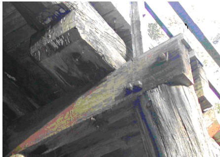
Figure 4: Load transfer by perpendicular to grain stresses
