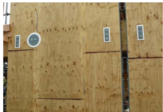
Figure 7. Shear walls showing the cylindrical shear connector with Teflon spacer, slotted location bolts, and U shaped yielding steel energy dissipaters
